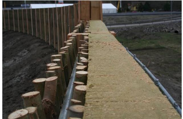
Birds eye view of barrier top showing woven panels, the noise absorbent core, and mesh panel.
