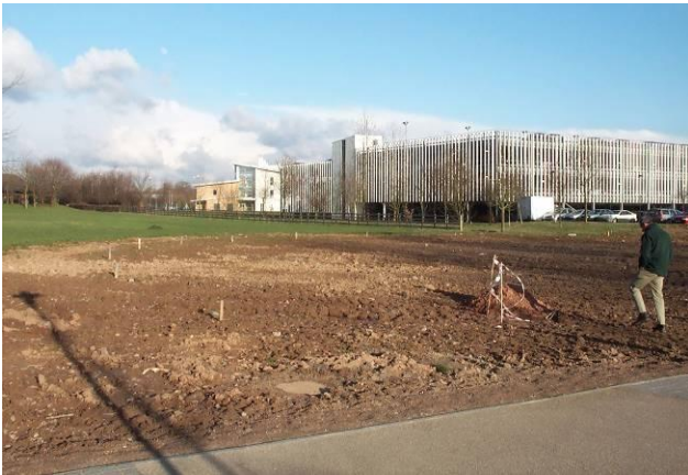
The site prior to the barrier being installed.
