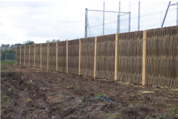
The finished construction prior to planting with climbers and evergreens.
