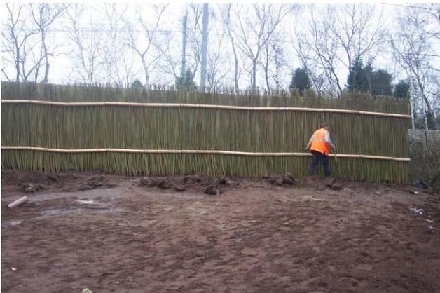
The installation of the acoustic Green Barrier in living Willow nearing completion.
