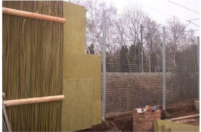
This barrier is constructed with one side living willow, a sound absorbing core, and the other side is metal security fencing.
