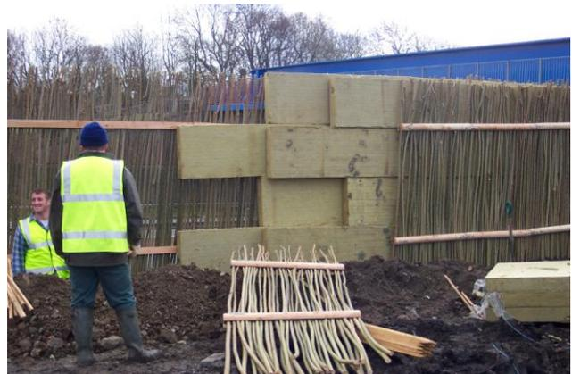
The Rock Delta core provides the sound absorption, giving an 11db reduction in noise.
