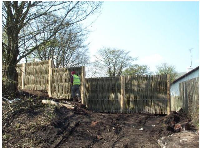
The Green Barrier can be planted up with climbers to further enhance the appearance. It has a life span of approx. 25 years.
