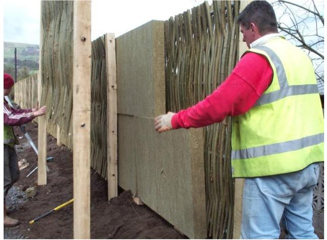
The RockDelta core has been tested to international standards and will absorb much of the traffic noise.
