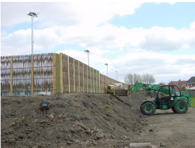
The Acoustic Green Barrier™ under construction
