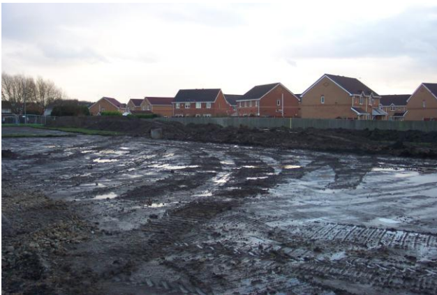
The site being prepared for the playing field
