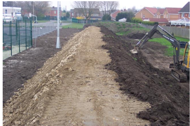
Building the 2500mm high bund
