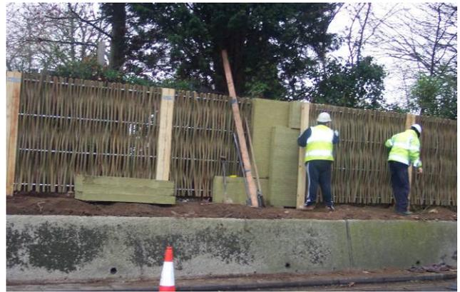
The acoustic insulation being installed and the facing panels erected.
