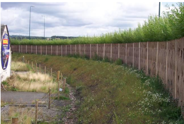
View of the woven side of the Green Barrier™ 3 months after installation.
