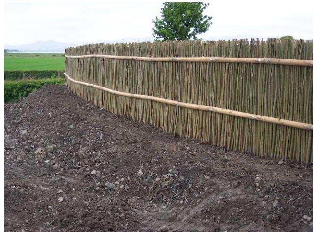
The Barrier under construction showing living side.
