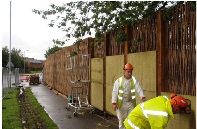
During construction, showing the noise absorbent core inserted between the woven willow panels.
