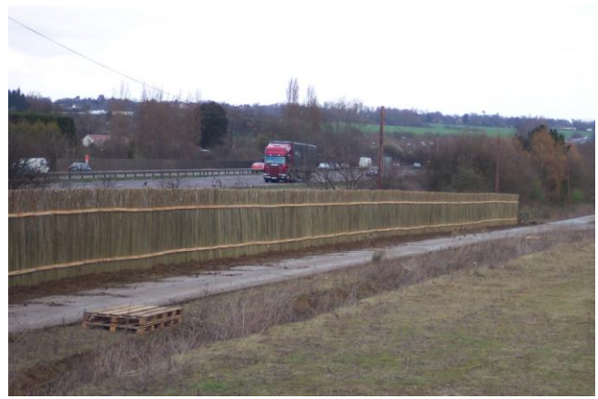
The Barrier is erected on a soil bund giving additional height and visible screening.
