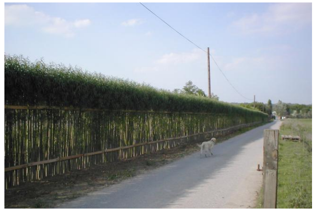
The completed Barrier, with irrigation system in place. Within a few weeks of installation the Barrier is already producing strong green side shoots and leaves.
