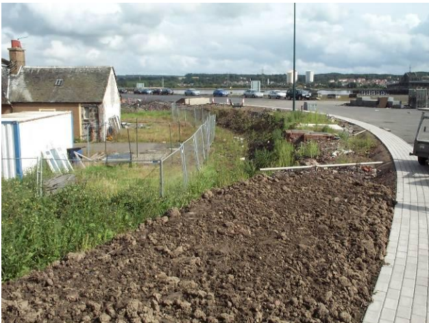
The site prior to installation of the Green Barrier™
